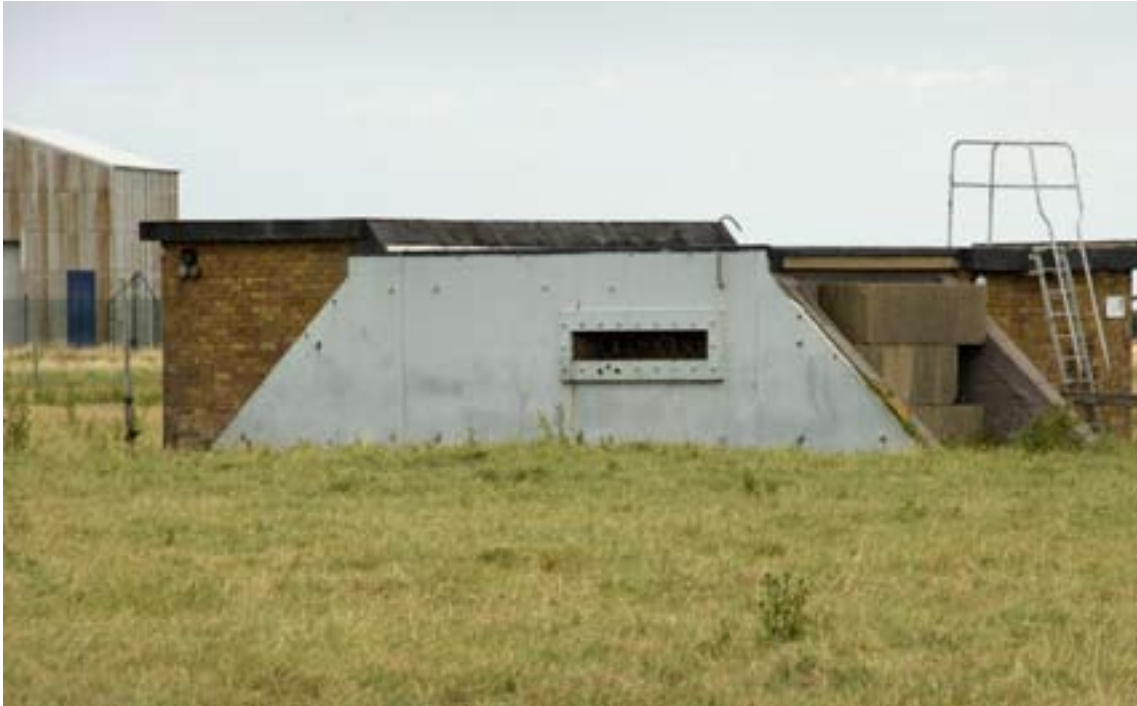
Figure 20: Fire Control Building J1. (c) English Heritage DP035952
