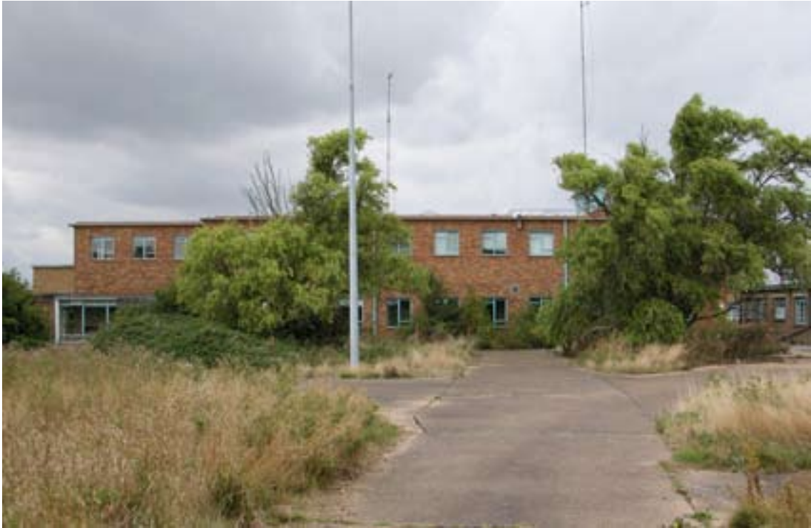
Figure 58: Administration Offices A6 built about 1955. (c) English Heritage
