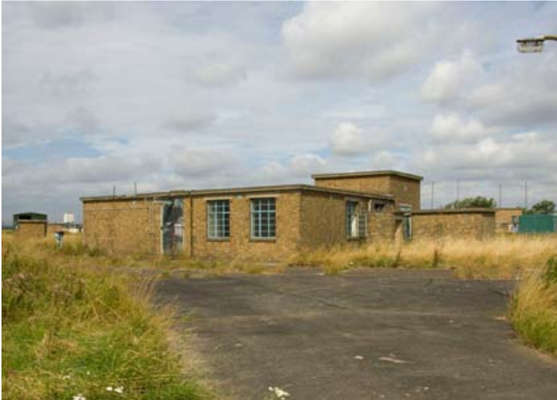
Figure 38 Explosives Preparation, Casting and Pressing X23, was 29, to the rear is the raised roof of the room that housed the 200 ton press. (c) English Heritage DP035935
