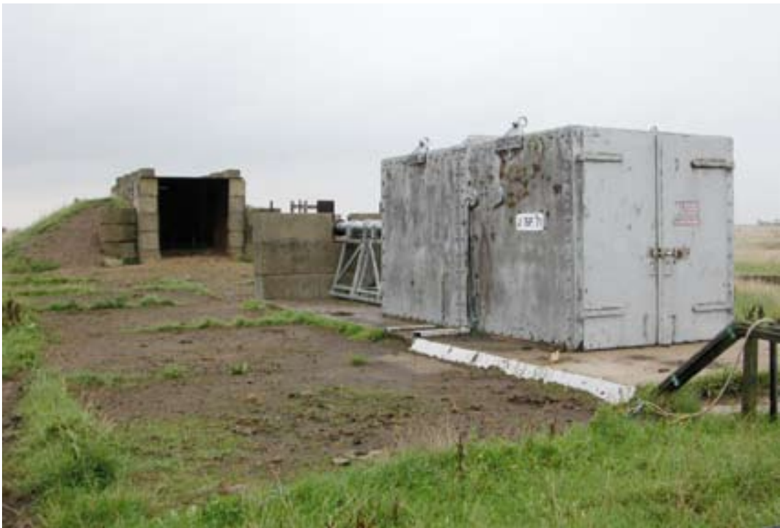
Figure 21 Compressed Air Launcher J/SF71, to the right is the steel container that housed the compressed air gun and to the left the Pendine block butt. (c) English Heritage
