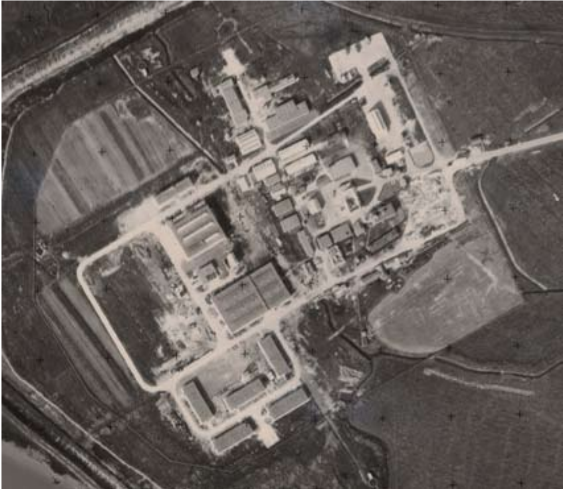
Figure 7: The Headquarters Area in July 1956 to the top are a series of pre-fabricated workshops and laboratories that were hastily erected after the decision to proceed with the H-bomb. RAF 58/2011 0084 27 July 1956 NMR (RAF) Photography
