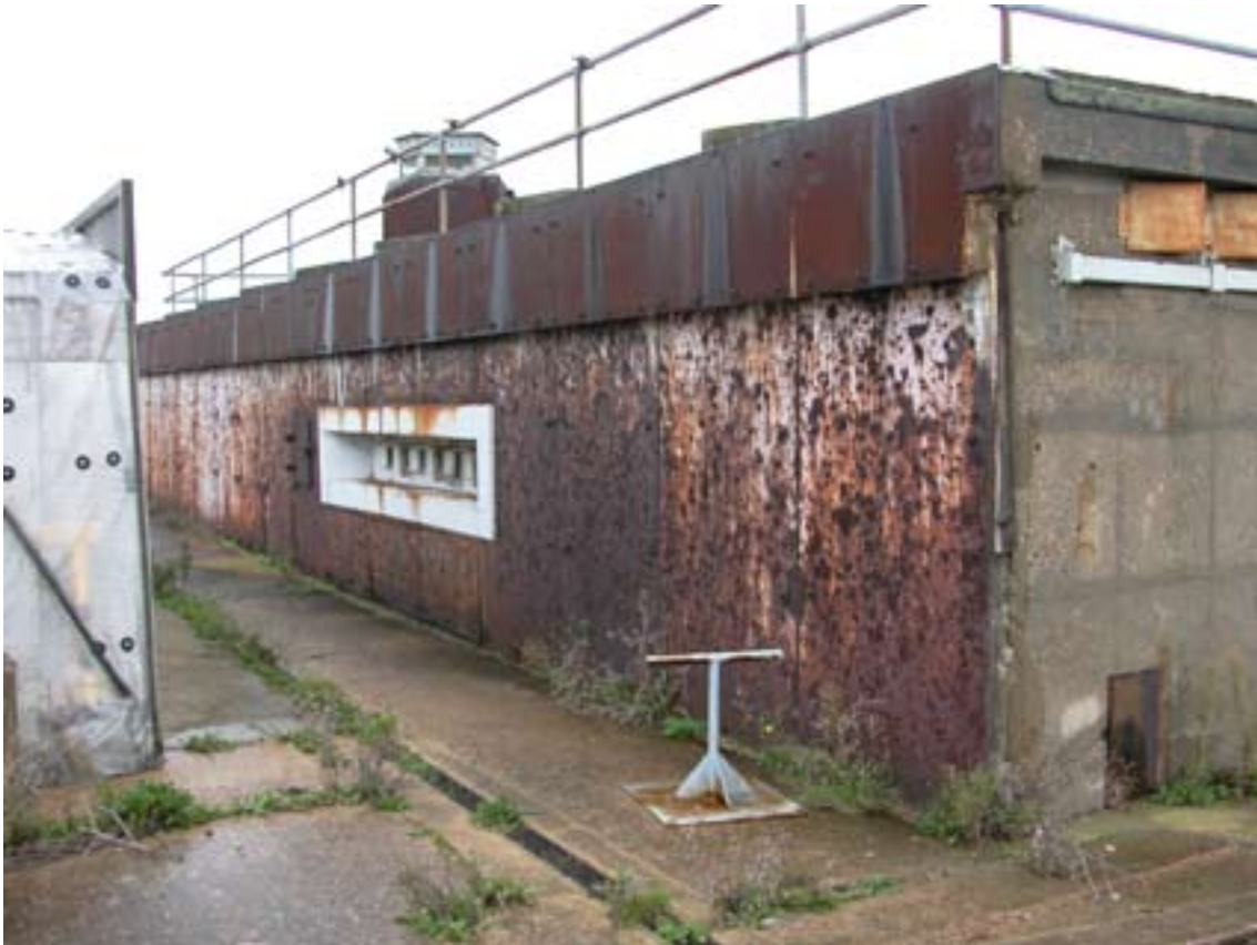
Figure 13: Fire Control Building and Instrumentation F4, showing the heavily pitted armoured steel wall facing the range, armoured observation apertures and roof turret. (c) English Heritage
