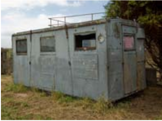
Figure 25: K13 Control Cabin, its aluminium body, sliding windows and mesh screens suggests it was probably a former overseas trials cabin. (c) English Heritage DP035972
