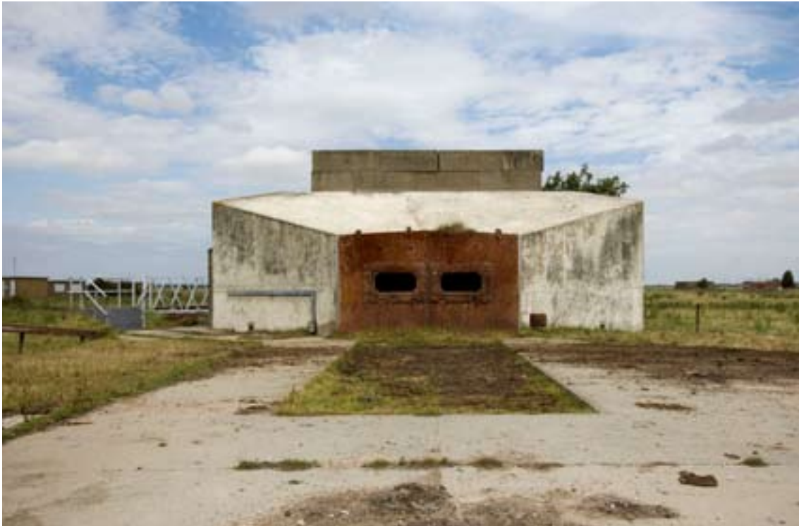
Figure 23: 1960s Instrumentation Building J10. (c) English Heritage DP035947
