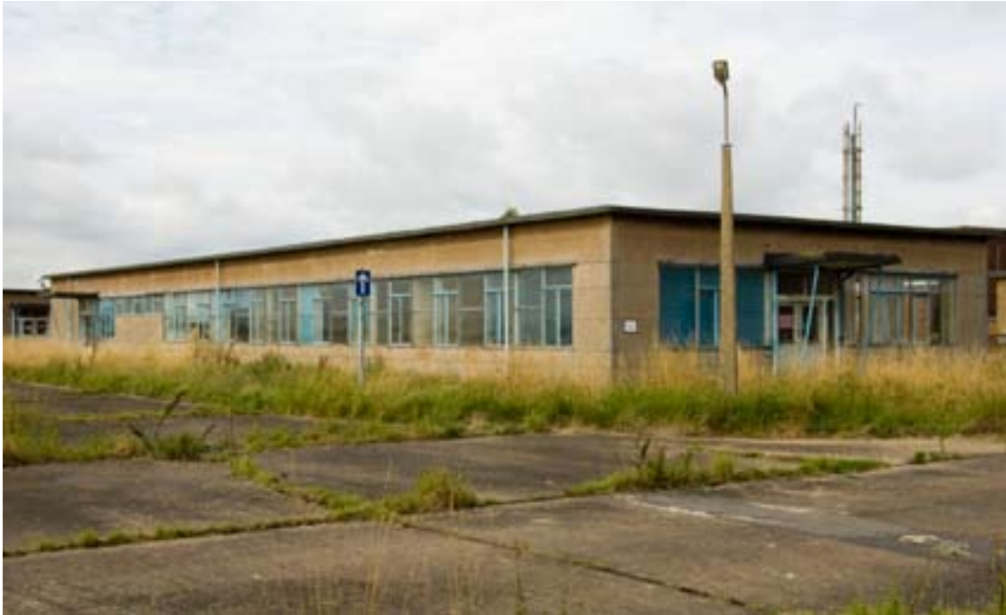
Figure 8: Laboratory LI was built in 1955 and illustrates many of the features typical of the mid-1950s pre-fabricated structures, including block panel wall construction, metal framed windows, and porch roofs supported by tubular steel arms. (c) English Heritage DP035968
