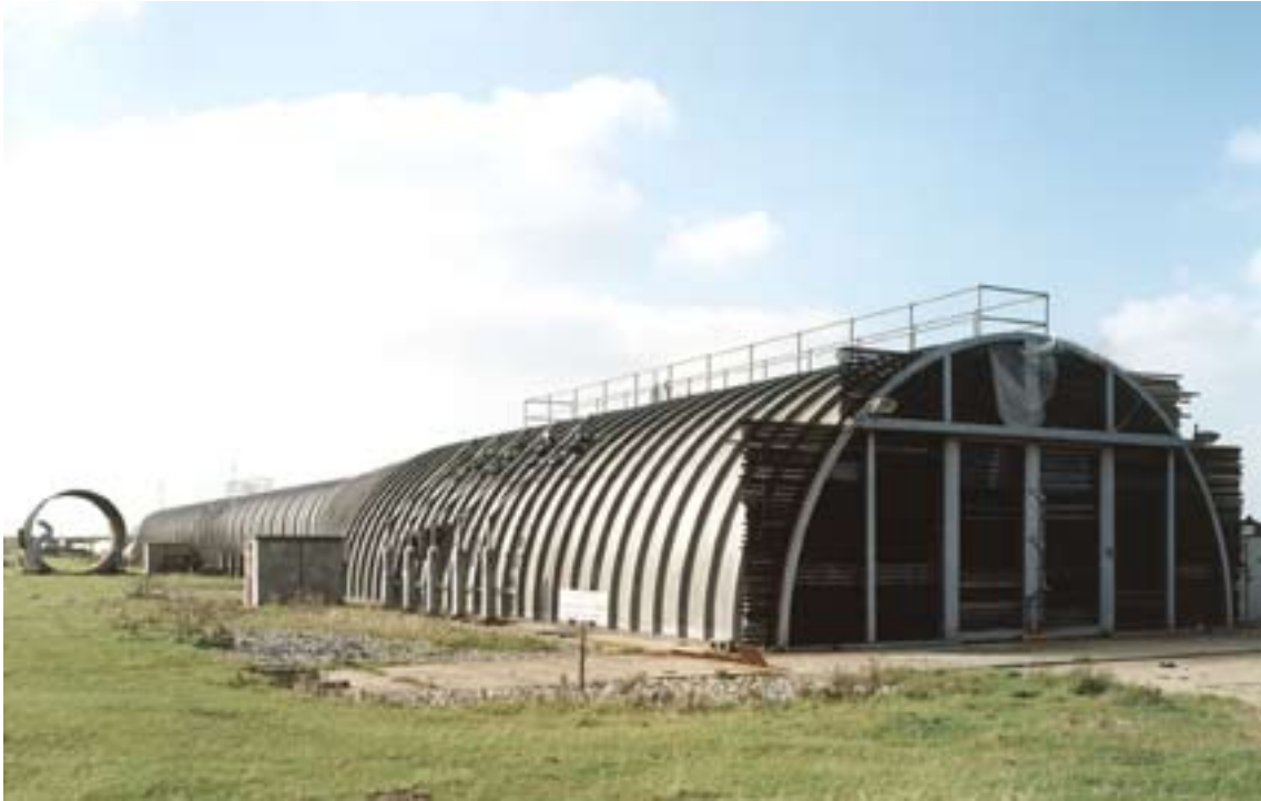
Figure 15: Mid 1960s Air Blast Simulator I/SF6. (c) English Heritage BB99/15990
