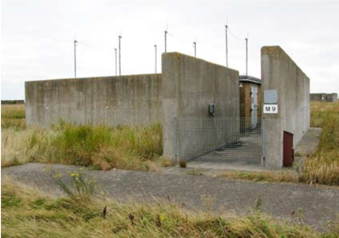
Figure 43: M9 Magazine, showing the typical protective L-shaped wall and inner brick magazine found in this area. (c) English Heritage
