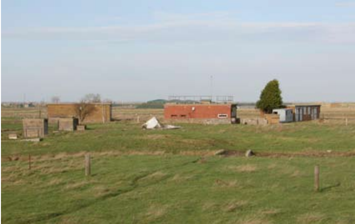
Figure 24: K site from its southern and range side, to the left is the Office and Instrumentation Building K4, in the centre the Very High Speed Recording Building K3 and to the right Range Support Workshop K2. (c) English Heritage
