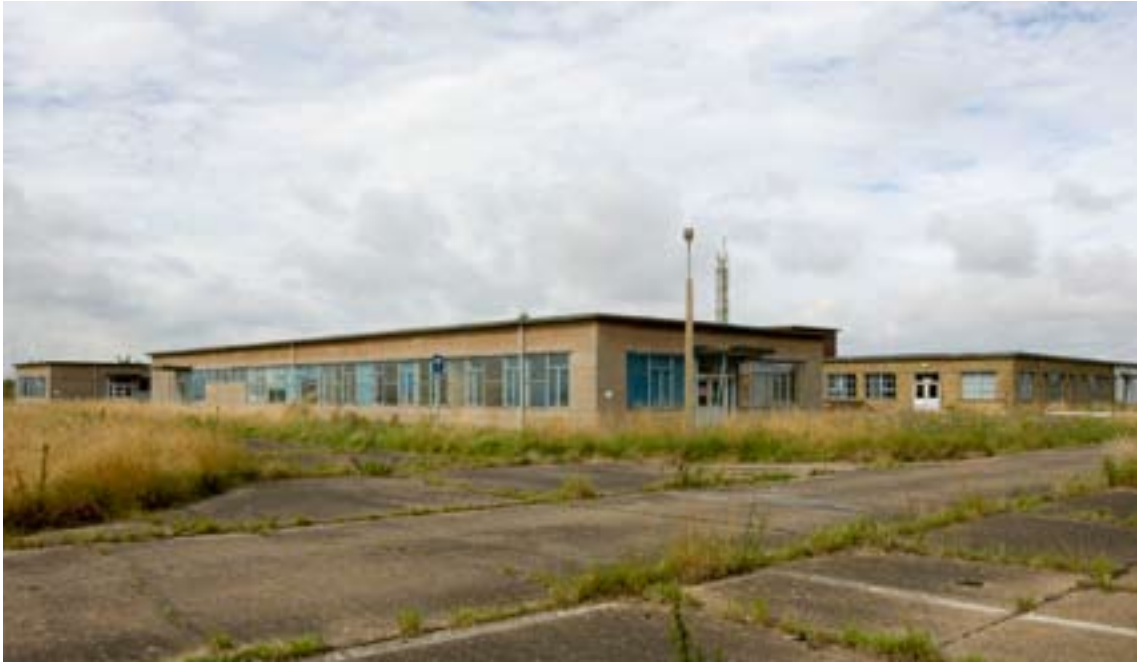
Figure 52: Prefabricated Laboratory L1 constructed about 1955 and to the right the slightly later brick built Electronics Laboratory L6. (c) English Heritage DP035967
