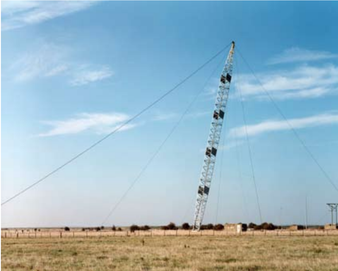
Figure 31: Spigot Intrusion Test Facility N/SF19. BB99/15977 (c) English Heritage
