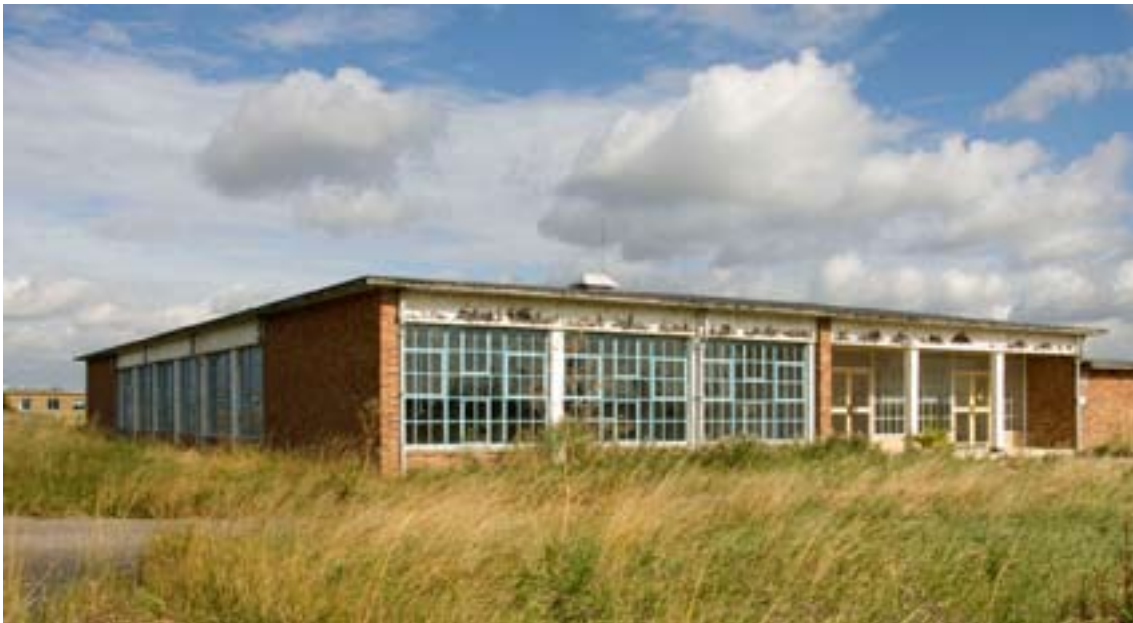
Figure 56: Canteen and Common Room A1, built in 1956. (C) English Heritage DP035913
