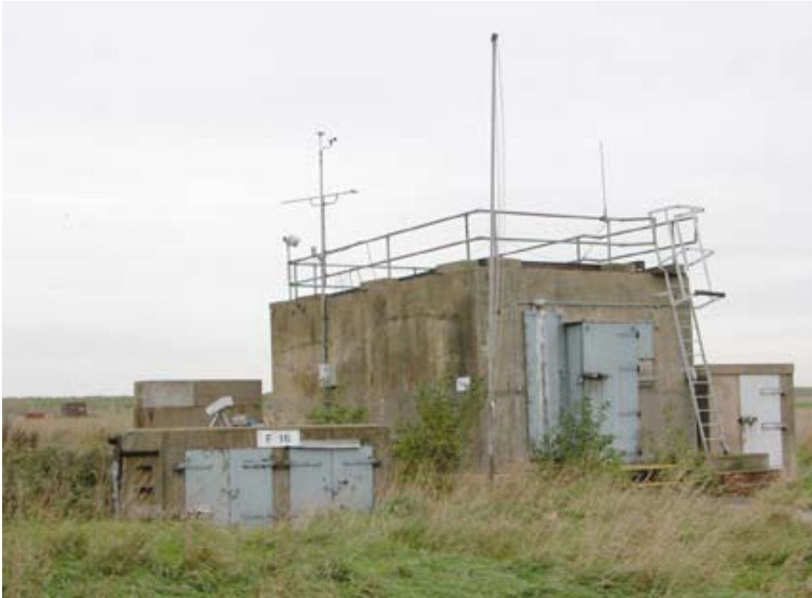
Figure 14: Fire Control and Instrumentation Building F6 and Cable Terminal Building F16. (c) English Heritage
