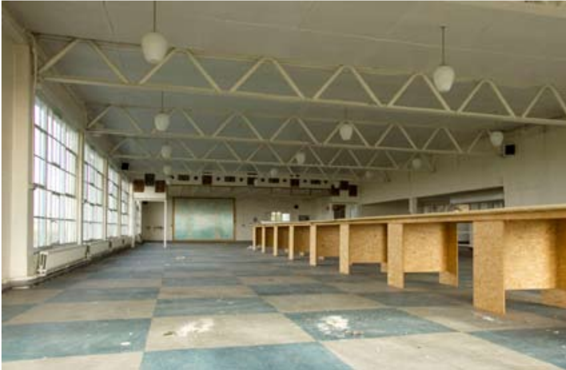
Figure 57: Canteen and Common Room A1, interior showing the main dining room with the bar to the rear. (C) English Heritage DP035914
